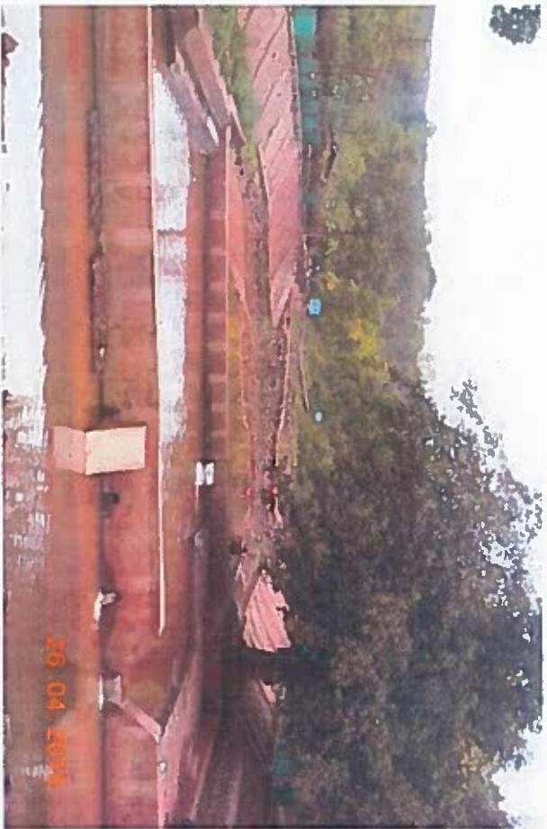
Photo – 5– showing the provision of check weir & check dam on the nallah
