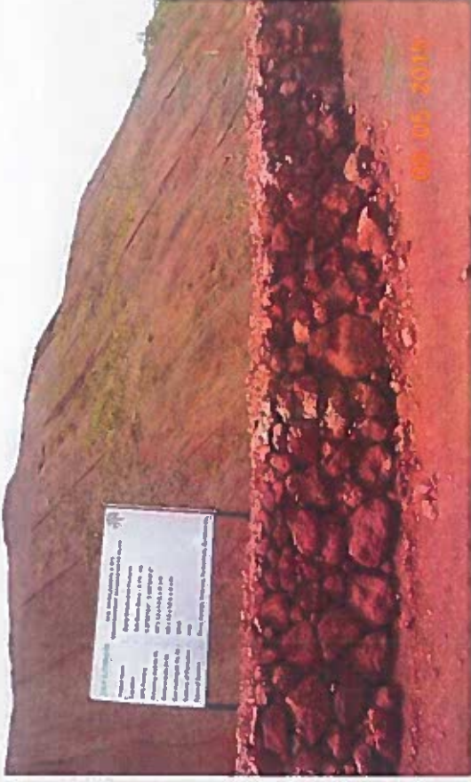
Photo – 2 - Showing the dump stabilization with coir mat application
