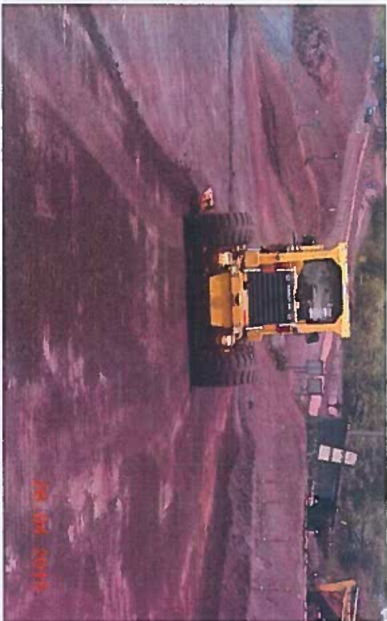
Photo – 12 – Showing the haul road maintenance with the help of grader
